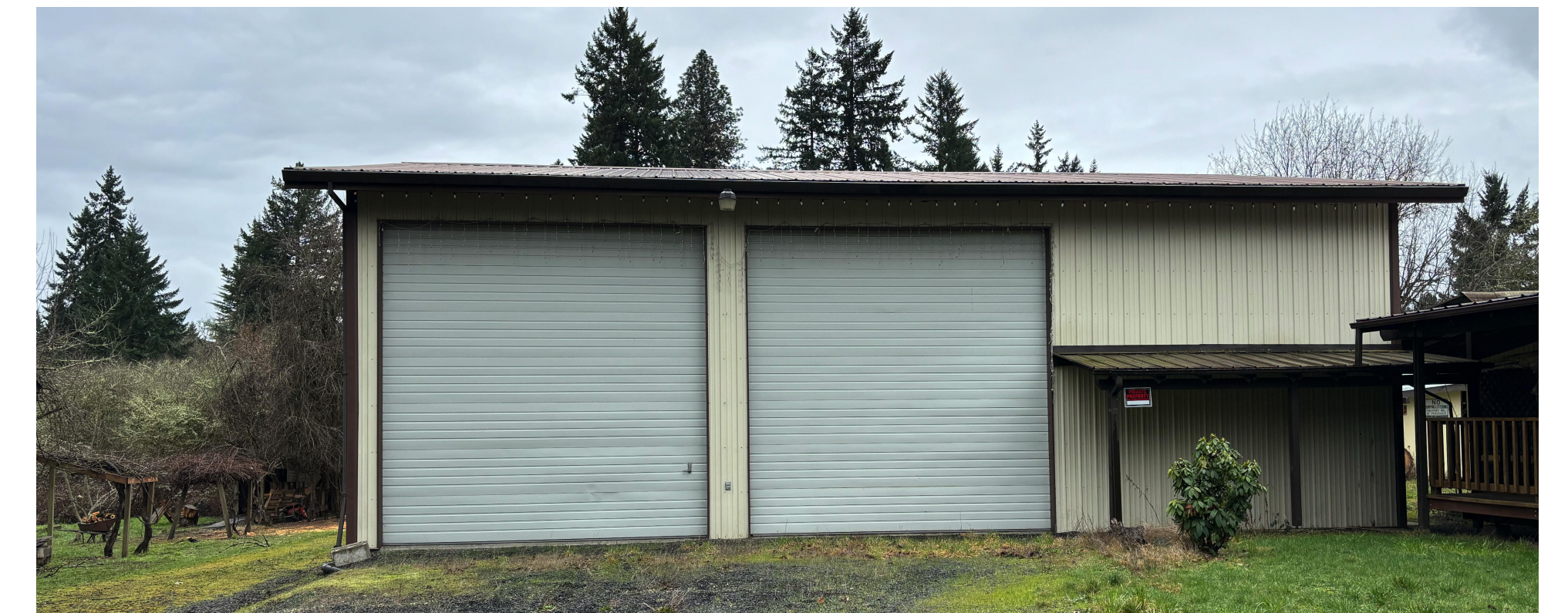
Shop Building New windows, located in existing garage door openings Existing siding to remain match existing as needed.
