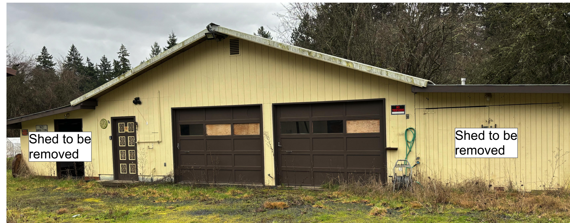
Garage Building - North Elevation New Bathrooms New Kitchen New horizontal lap siding New doors and windows located in existing garage openings.
